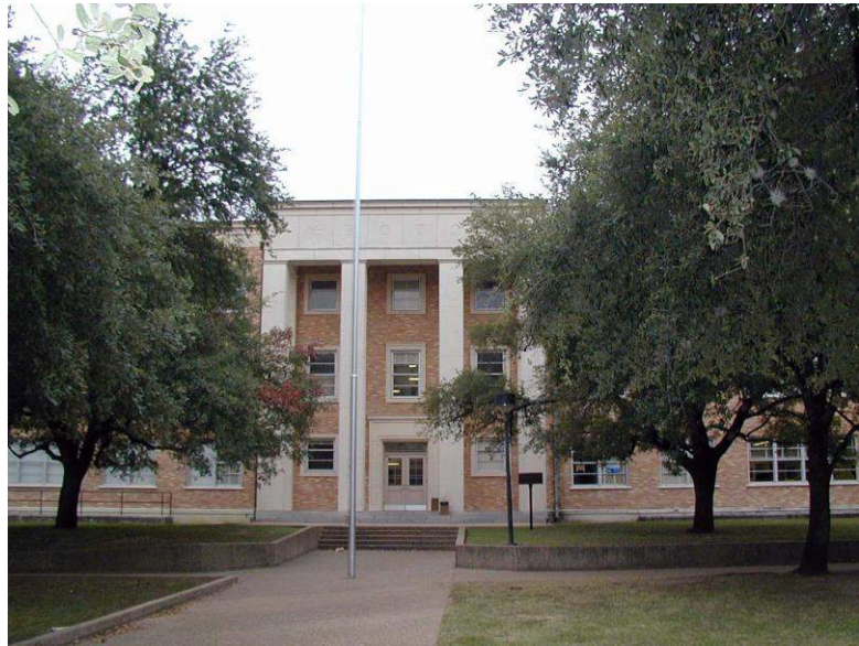
ROTC Building on the East Mall, later renamed Russell A. Steindam Hall
