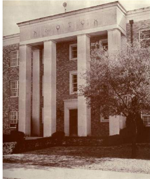
East Mall Entry for the ROTC Building
